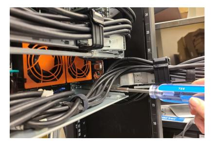
**Step 10:** Install the lower brackets onto the CMA tray.
