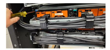
**b.** Swing the CMA crossbar and CMA arm(s) to the side and out of the way.
